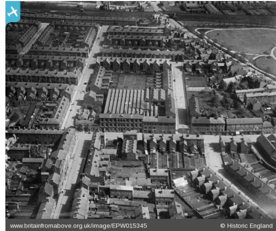
Aerial photograph showing Britannia Mill (centre) facing Payne’s Lane. Running alongside the factory site is Britannia Street, with the Binley Oak on the corner. Gosford Green is visible in upper right corner.
